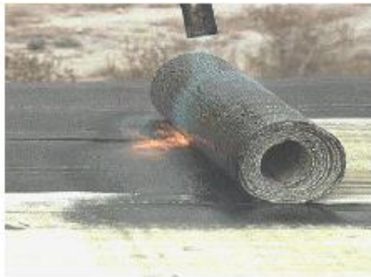
Modified Bitumen Roof [RFG BI]
